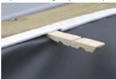
Figure 22 – Blocking the liner in position using half clothes pegs
