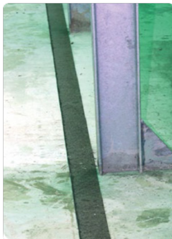
Figure 6 – Laying the bituminous strips
