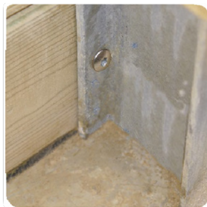
Figure 8 – Fastening the slats to the supporting braces
